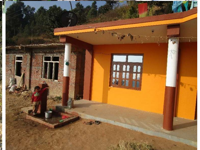
Picture 3: “one house, one tap” project in Chhange WSS has improved the quality of life of the community
