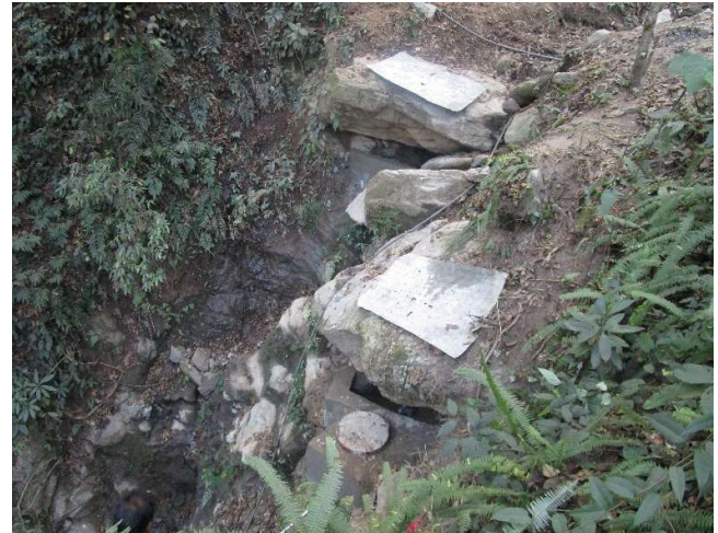
Improved intake with gravel packing and valve box
