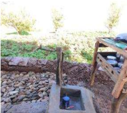
Her tap under maintenance with meter box
